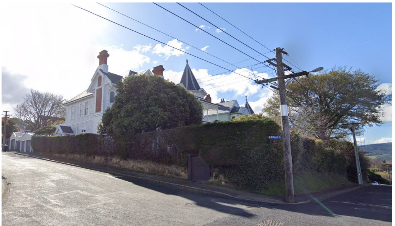
Figure 2. View of T454 from corner of Tweed and Fifield Street, facing north.
