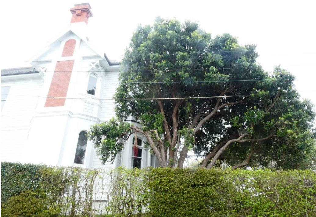
Figure 2. View towards T454 from south of the site on Fifield St.
