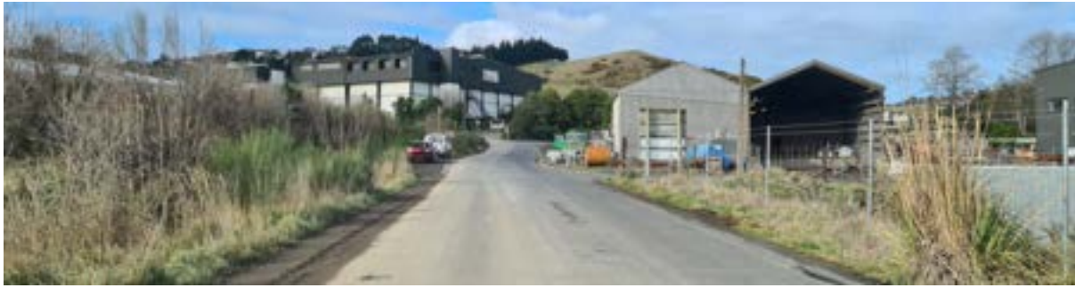
Kaikorai Valley Road looking north showing the intersection with McLeods and Eclipse Roads
