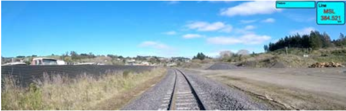
McLeods Road Private looking south-west showing entrance to Nash & Ross facility and existing bridge structures over the Kaikorai Stream at the eastern side of the facility.
