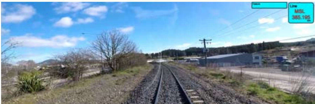
Rail Corridor - MSL 385.145 looking west showing existing bridge at end of Boomer Street private
