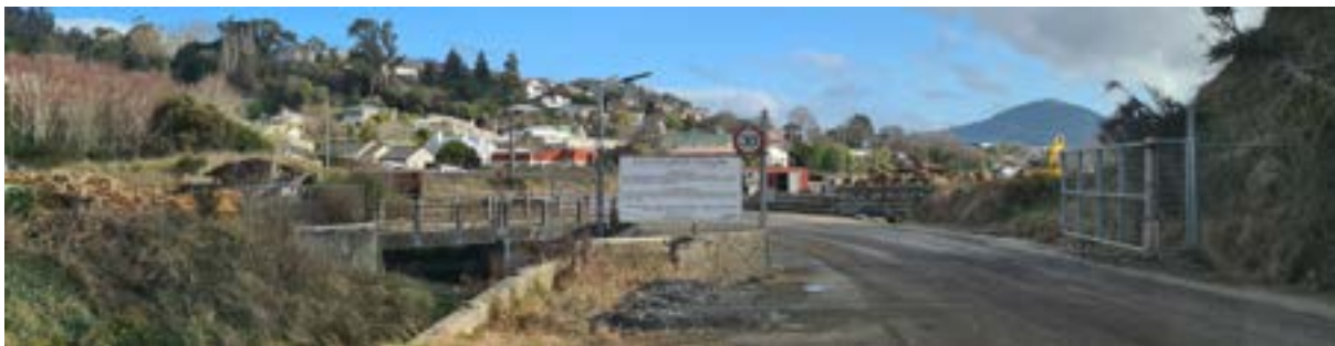
McLeod Road at Kaikorai Valley Stream looking north-east along the historical rail corridor
