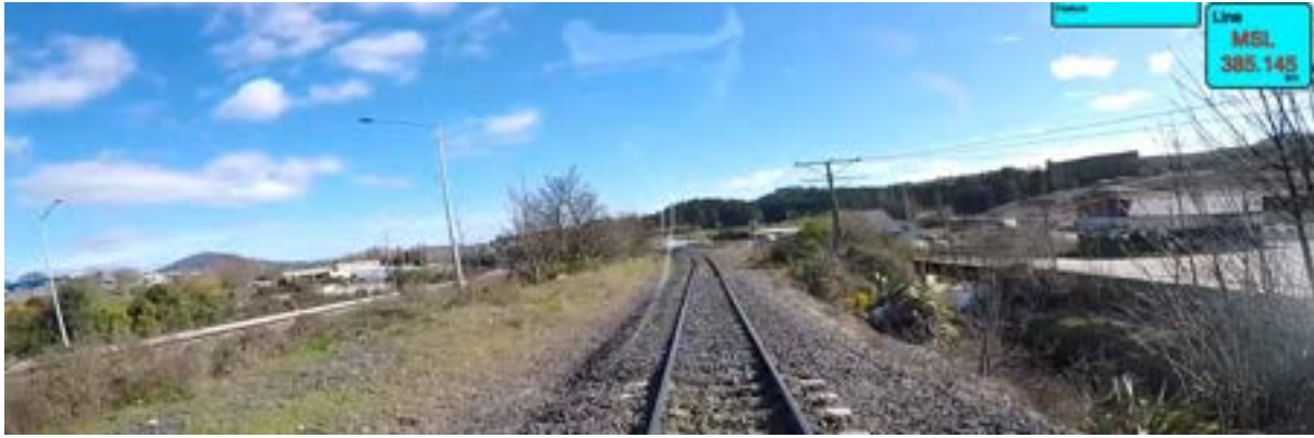
Rail Corridor - MSL 385.016 looking west showing Nash & Ross facility interface with Kaikorai Stream
