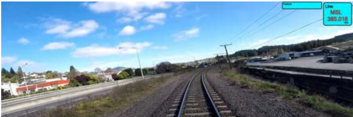
Rail Corridor – MSL 384.669 looking west
