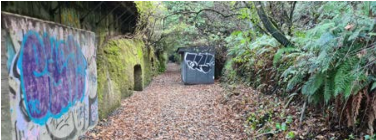
Caversham Tunnel entrance track looking west from SH1 north side shared path
