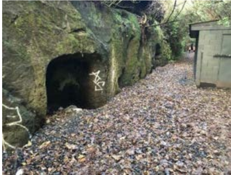
Figure 6-5: Trail route north of Caversham Tunnel
