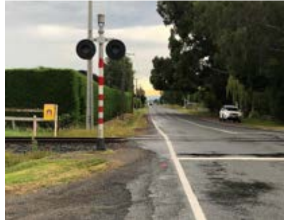
Figure 3-2: southside of crossing
