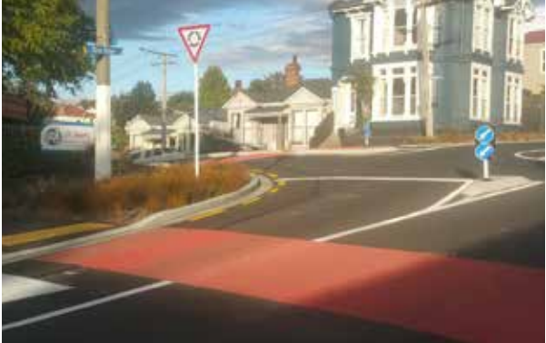
Permanent kerb buildout at intersection
