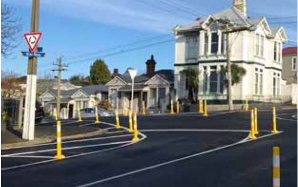
Trial kerb buildout at intersection
