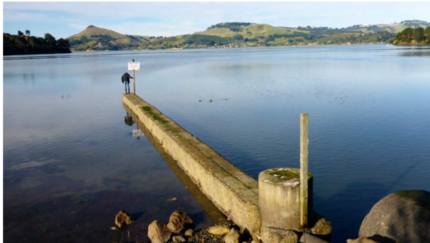
Figure 16. The extended pipe that conveys overflow wastewater and stormwater into Sawyers Bay.
