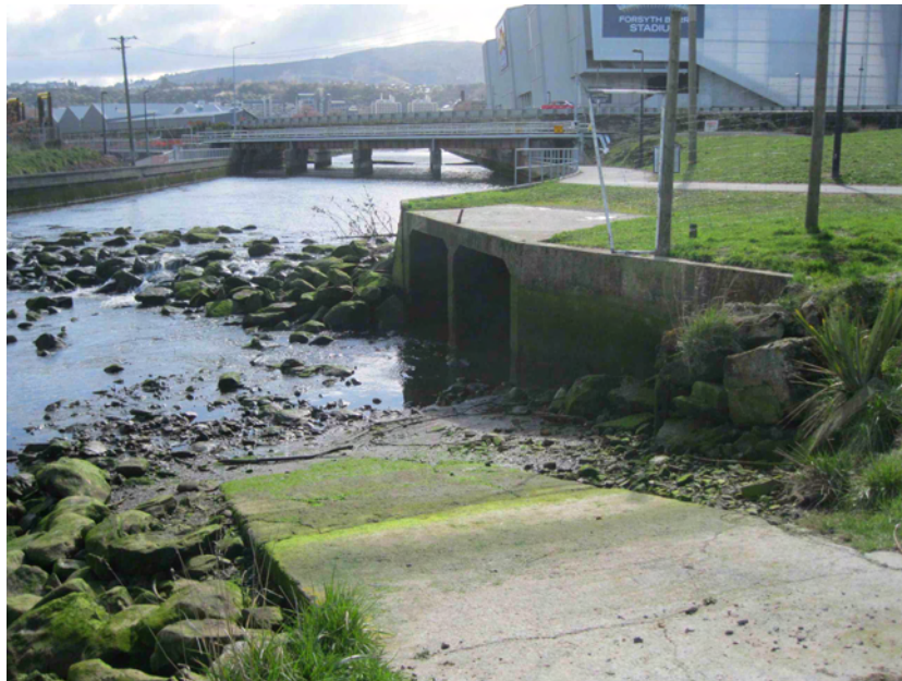
Figure 9. Photo of lower Water of Leith showing the conduit that discharges Butts Creek and stormwater that may carry wastewater from the Harbour Terrace / Union Street East overflow site.
