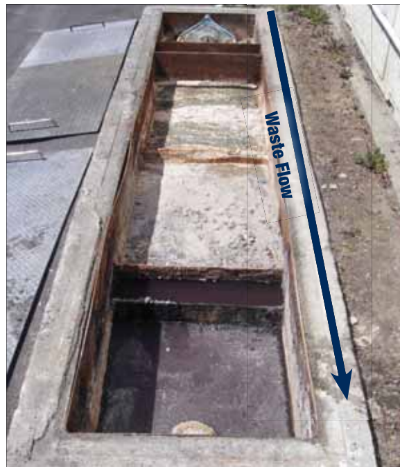
Fully Effective Grease Trap Just Before Cleaning
