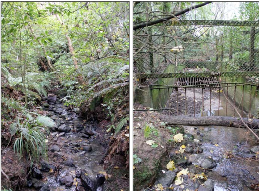
Figure 5-7: Mason Street 2 Downstream - Left: Assessment Site Lower Reaches; Right: Location of Entry to Stormwater Pipes
