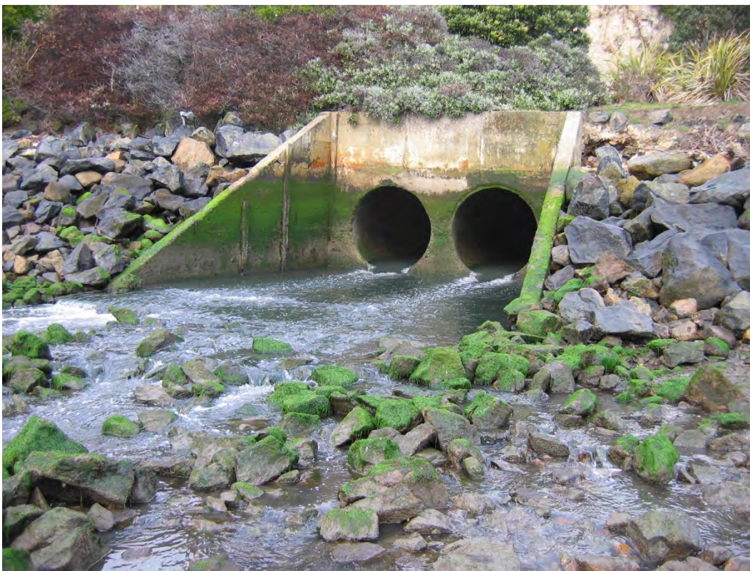
Figure 5-1: Portobello Pump Station Outfall
