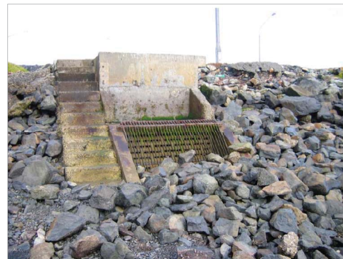
Harbour Outfall Structure at Teviot Street
