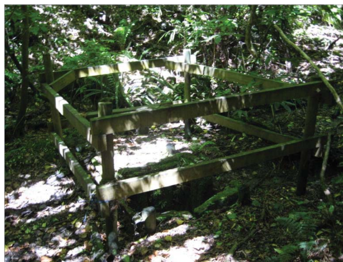
Ajax Road Intake
