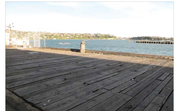
Fryatt Street Wharf
