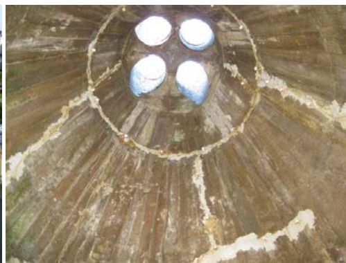
Bell Chamber Outfall Ceiling
