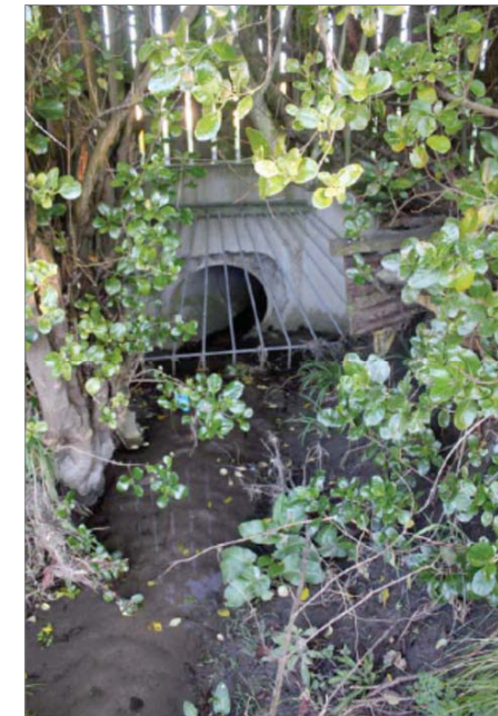
Culvert Intake at 71 Tahuna Road
