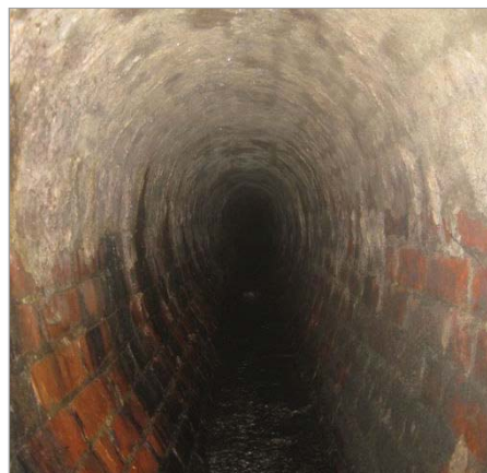
Brick Arch Stormwater Pipe on Hanover Street
