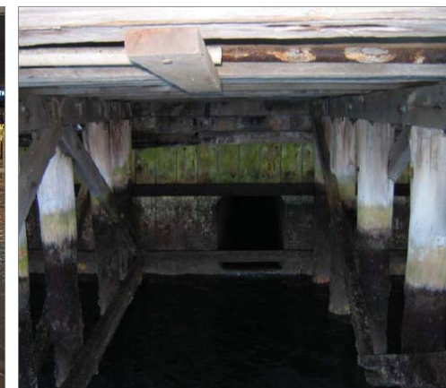
Catchment Harbour Outfall at Bauchop Street
