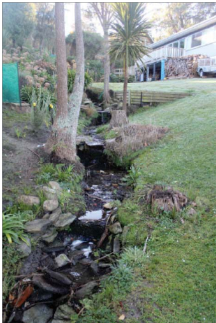
Open Channel at Top of Chisholm Place
