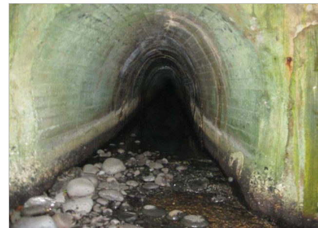
Outfall Pipe to Bell Chamber at Second Beach
