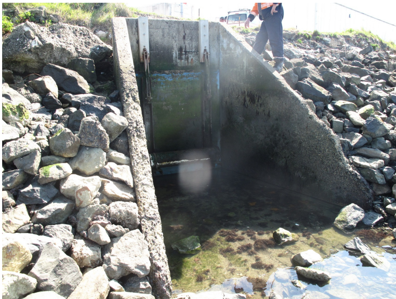
Figure 5-1: Main Kitchener Street Stormwater Catchment Outfall
