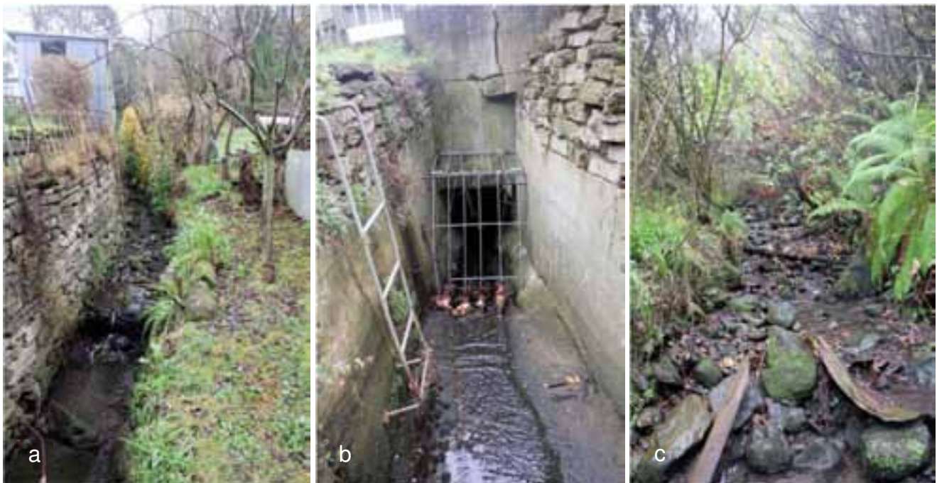
Figure 5-8: Orari Street 4 Stream Assessment Sites – (a) Upstream; (b) Entrance to Stormwater Pipes near Upstream Site; and (c) Downstream
