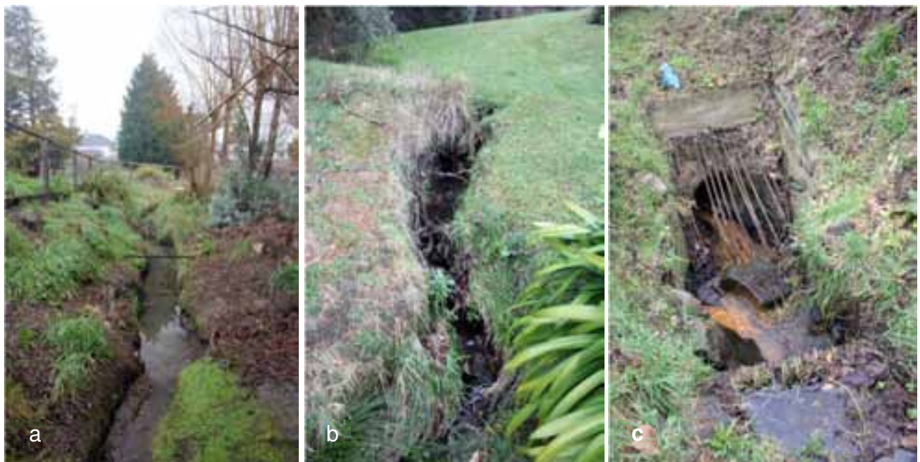
Figure 5-5: Orari Street 1 Stream Assessment Sites – (a) Upstream; (b) Downstream; and (c) Entrance to Stormwater Pipes near Downstream Site
