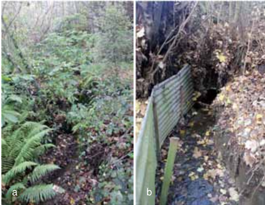
Figure 5-6: Orari Street 2 Stream – (a) Assessment Site; and (b) Entrance to Stormwater Pipes
