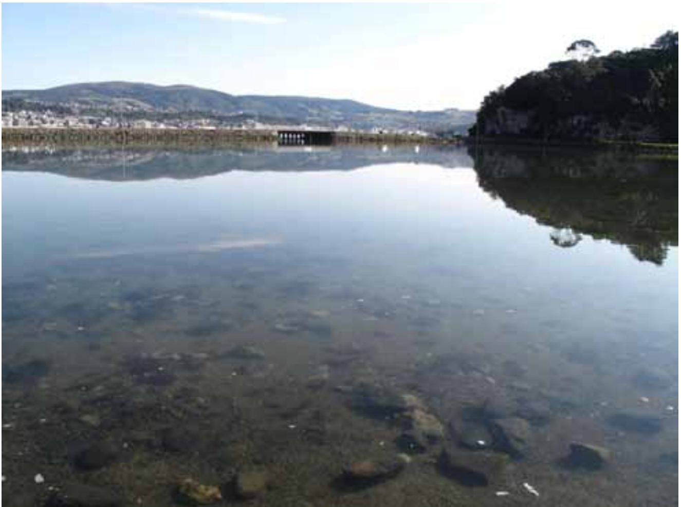
Figure 5-2: Andersons Bay Inlet, showing Discharge to Otago Harbour beneath the Portobello Road Causeway
