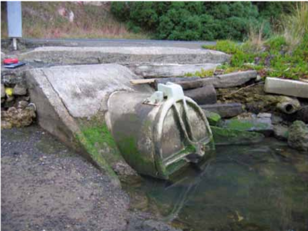
Figure 5-1: Shore Street Catchment Outfall (Andersons Bay Inlet)
