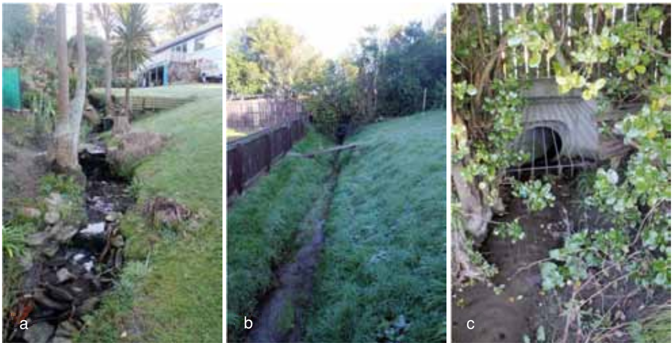
Figure 5-6: Shore Street 1 Stream Assessment Sites – (a) Upstream; (b) Downstream; and (c) Entrance to Stormwater Pipes near Downstream Site
