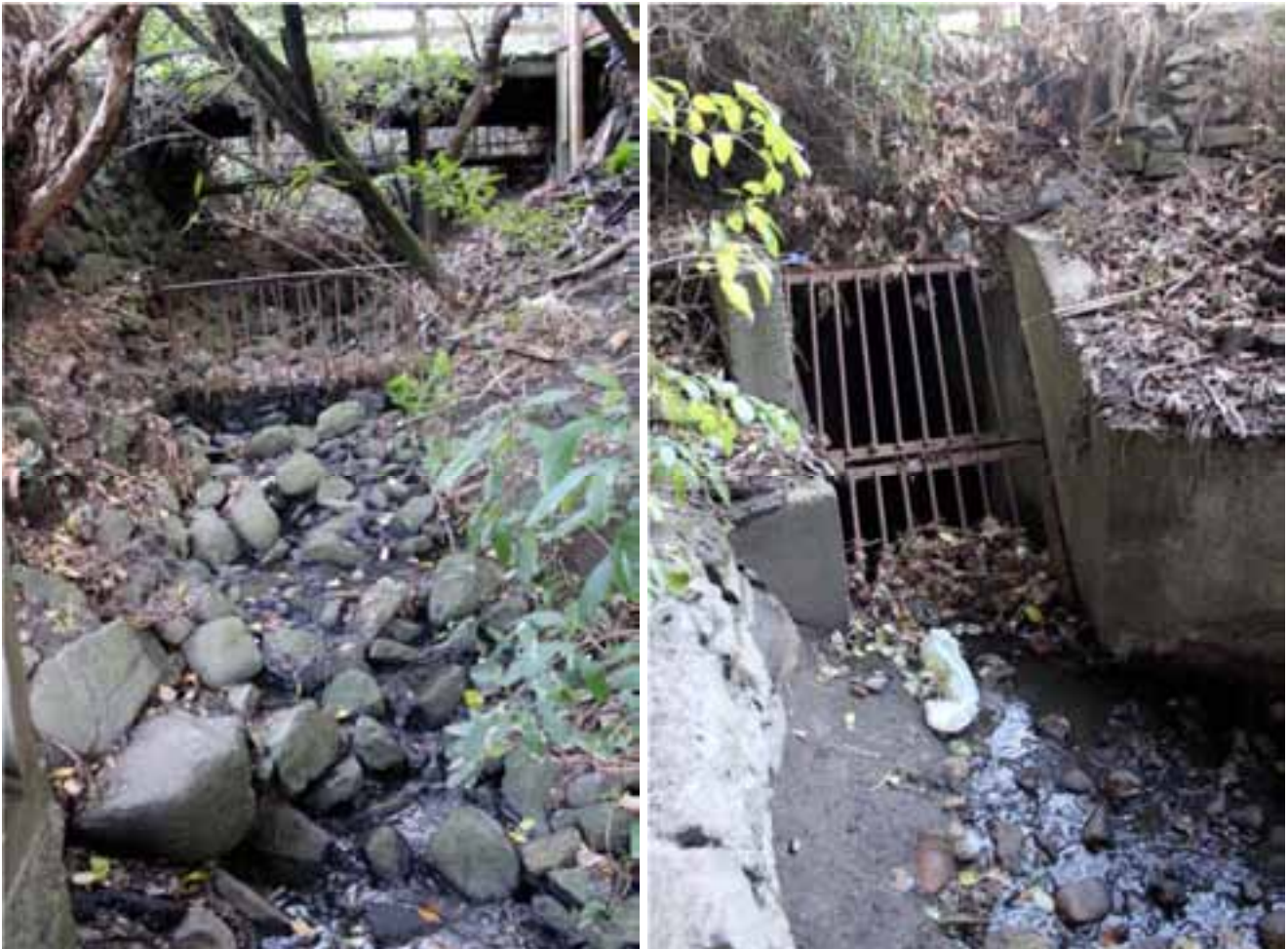
Figure 5-6: St Clair 2 – Left: Assessment Site; Right: Entrance to Stormwater Pipes at Downstream End of Site
