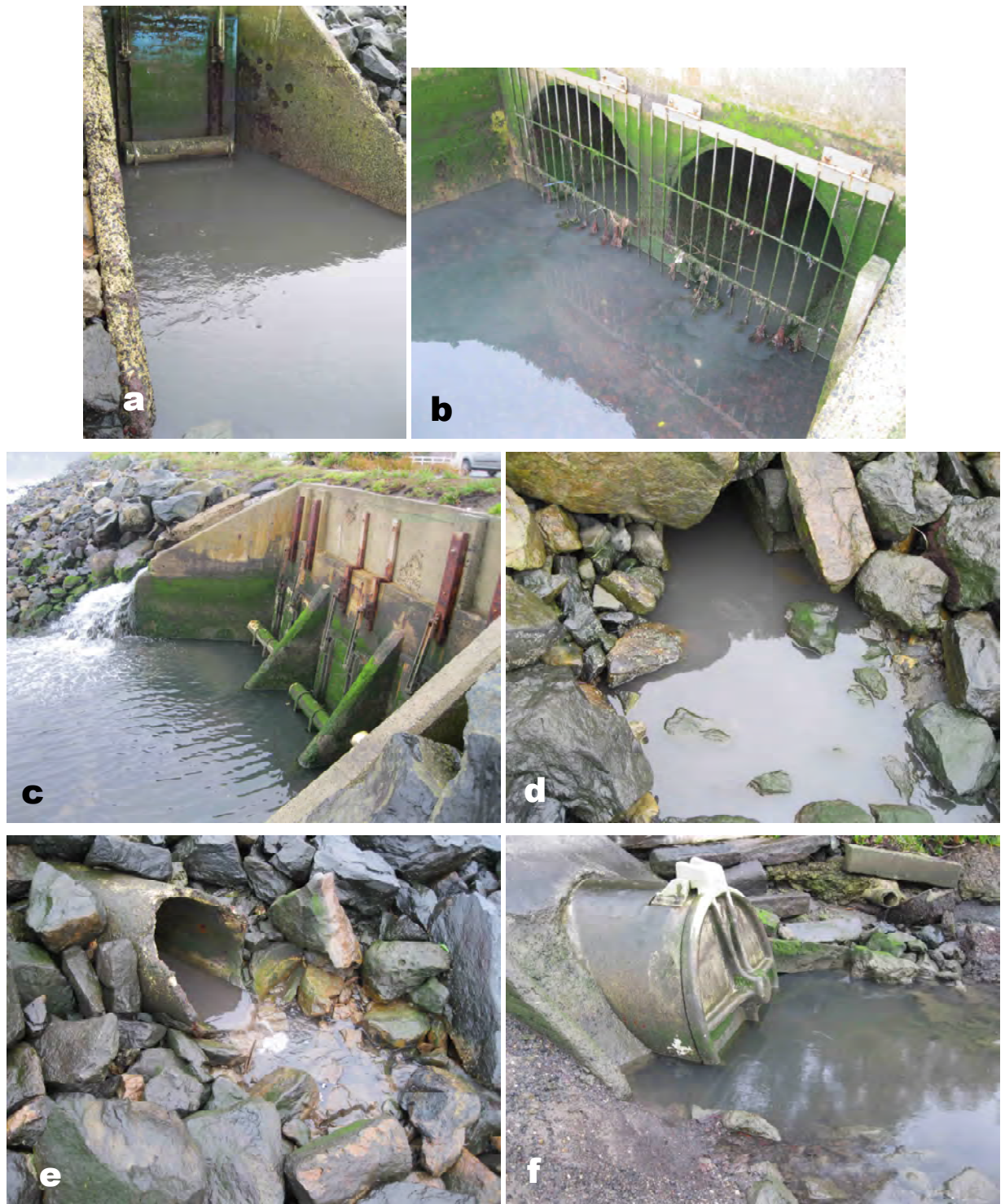
Figure 3 Discoloured stormwater discharging from (a) Kitchener Street; (b) Portobello Road; (c) Orari Street; (d) Midland Street; (e) Teviot Street; and (f) Shore Street.
