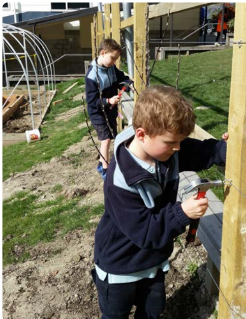
Building the fence above the garden
