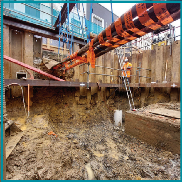
The lower Stuart Street works involved digging a large excavation five metres deep, in order to unearth historical pipes dating back as far as 1887. Cover image: Aerial photo of The Octagon in 1955.
