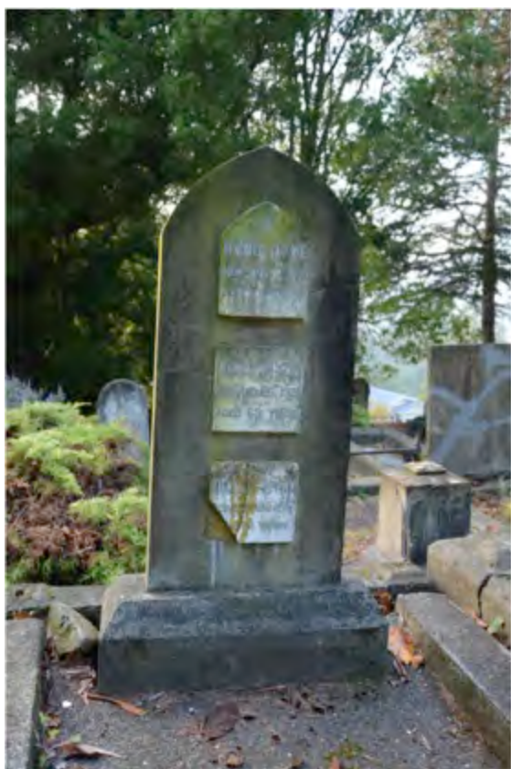
Left: cast concrete plate with marble panels fitted
